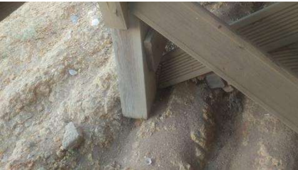
Image 112: This image shows one of the main supports for this staircase which is not fixed due to erosion. It is only a matter of time until collapse and potential visitor injury or death.
