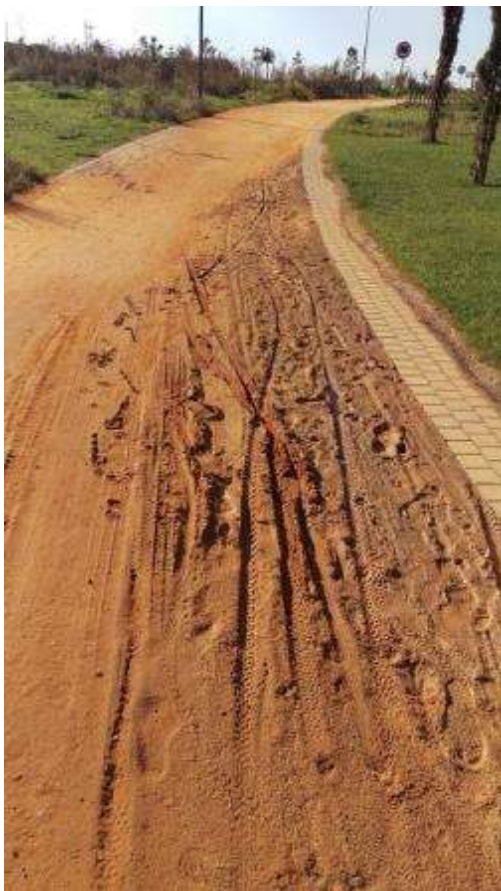
Image 83: Trail surface at Parque Ribeirinho de Faro that has deteriorated due to over-spraying from irrigation system
