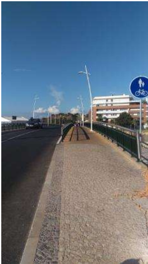
Image 100: Bridge at Lagos showing best-practice segregation of road and cycle/pedestrian traffic. This could be replicated at Praia do Faro, see image 91
